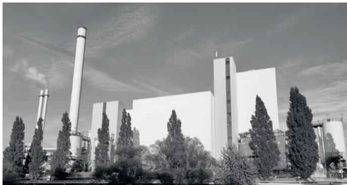
Abb. 1 Waste generation plant, Hamburg
