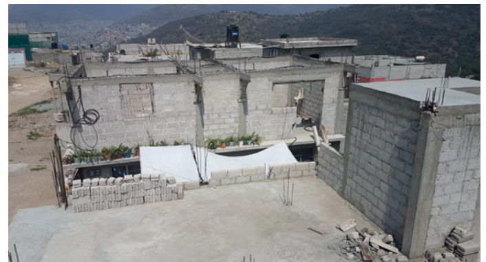
Abb. 2 Construction site of self-built home, Ecatepec, Mexico City Metropolitan Area
