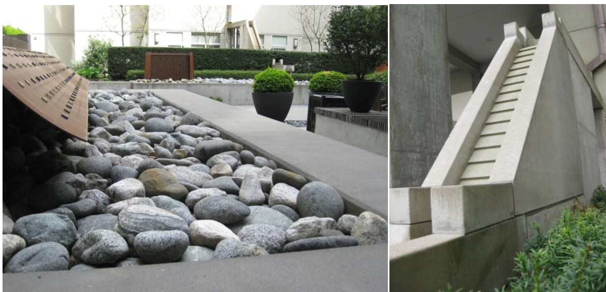
Fig. 71. Water from the roof tops splashes over sculptural cascades and Cor-Ten steel weirs before it disappears between river stones (© J. Hoyer).
