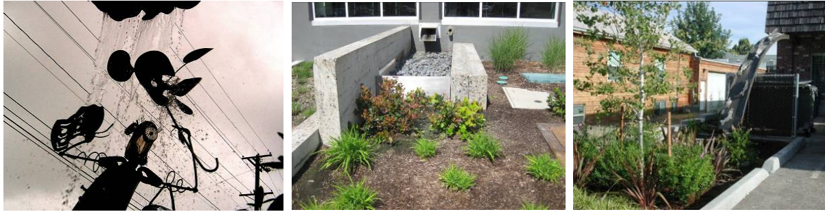
Fig. 20. Portland encourages citizens to disconnect their downspouts (middle). Butler promotions (left) and new seasons market (right) did it in an artistic manner (© J. Hoyer (middle), © Bureau of Environmental Services, City of Portland Oregon, USA (left and right)).
