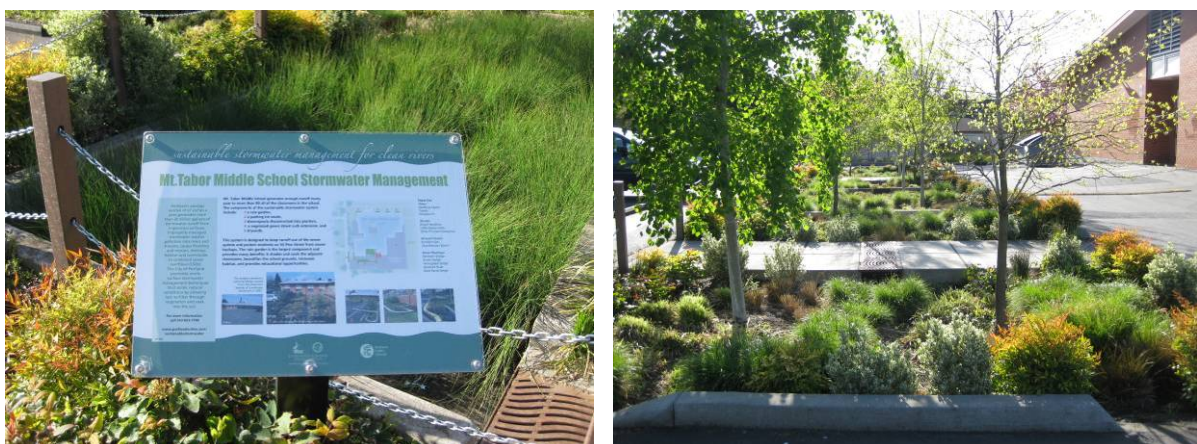
Fig. 21. Rain garden and infiltration planter at Mt. Tabor Middle School: Children of the school are educated about the advantages of decentralised stormwater management and a pilot project on the school yard shows how it can look like (© J. Hoyer).
