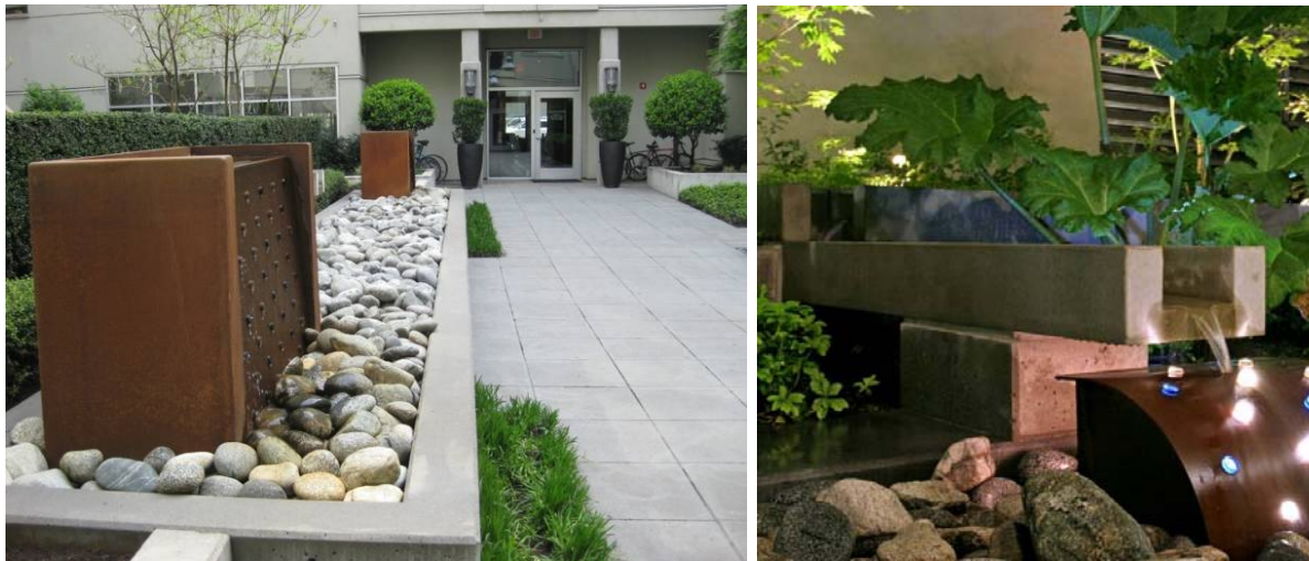
Left: Fig. 72. Cor-Ten steel fountains; Fountains only function when the cistern is filled; At night, fountains are lit from inside (© J. Hoyer); Right: Fig. 73. The best time to visit the courtyard is at night and when it is raining (© Koch Landscape Architecture).
