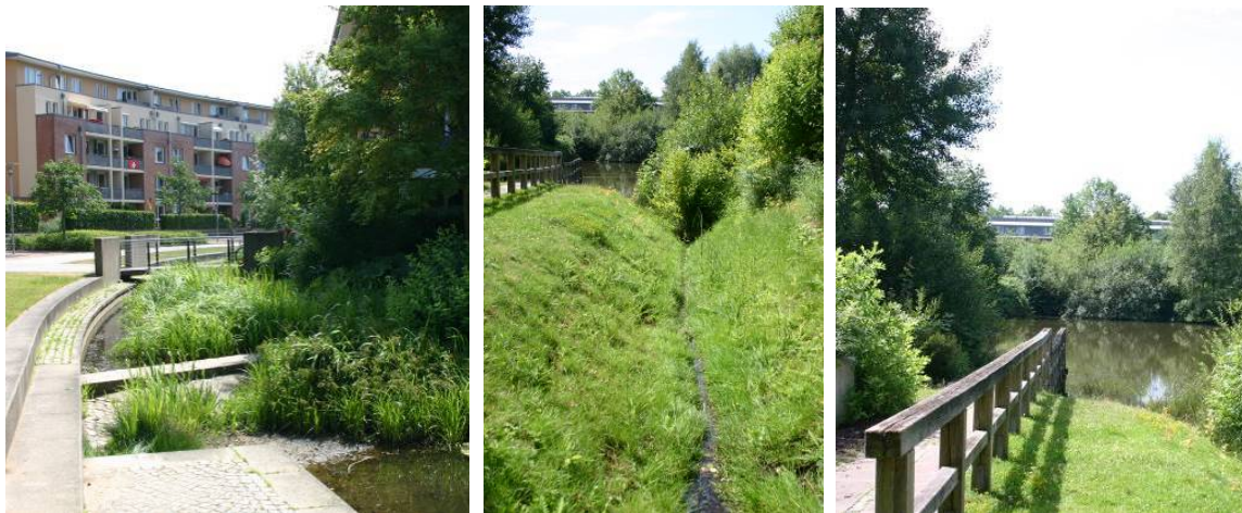
Fig. 45. Water is collected in channels and swales and led to centrally located retention ponds (© M. Derneden).
