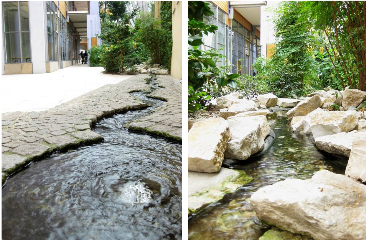
Fig. 82 & 83. A water course, which is artificially shaped at the beginning and then turns into a nature-oriented design, uses rainwater collected in the underground cistern (© J. Hoyer).
