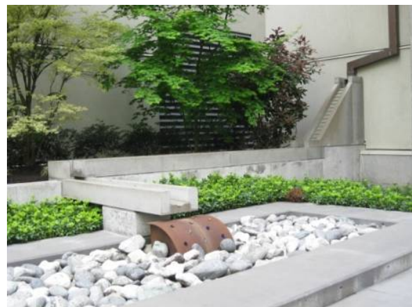
Left: Fig. 69. Central seating area with wooden furniture and plant pots (© J. Hoyer). Right: Fig. 70. One of the 3 cascades leading stormwater from the roof to detention basins filled with riverbed stones (© J. Hoyer).
